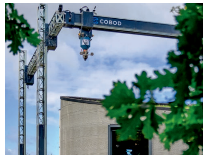
The low-energy house has functional furnishings (above left) and can be used in a variety of ways. The additive technique used produces walls with a visually appealing design (above right). In the construction effort, Europe's largest 3D concrete printer was used (left).
